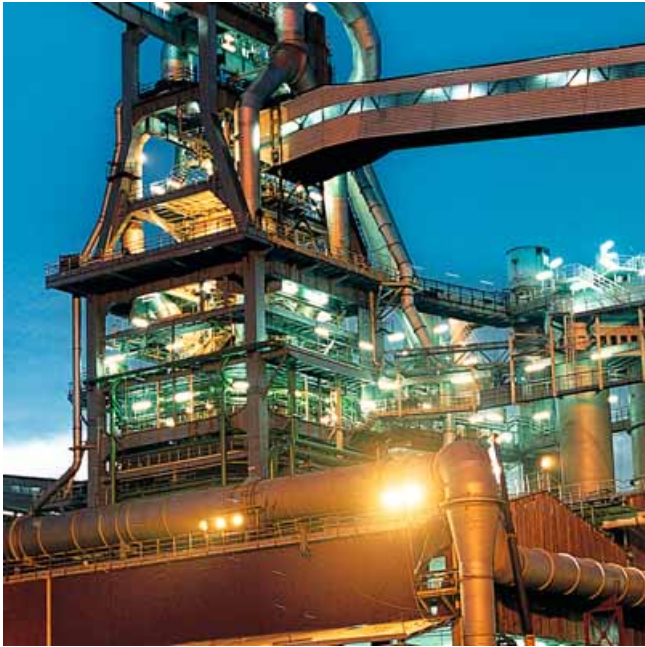
Industrial application: Refinery
